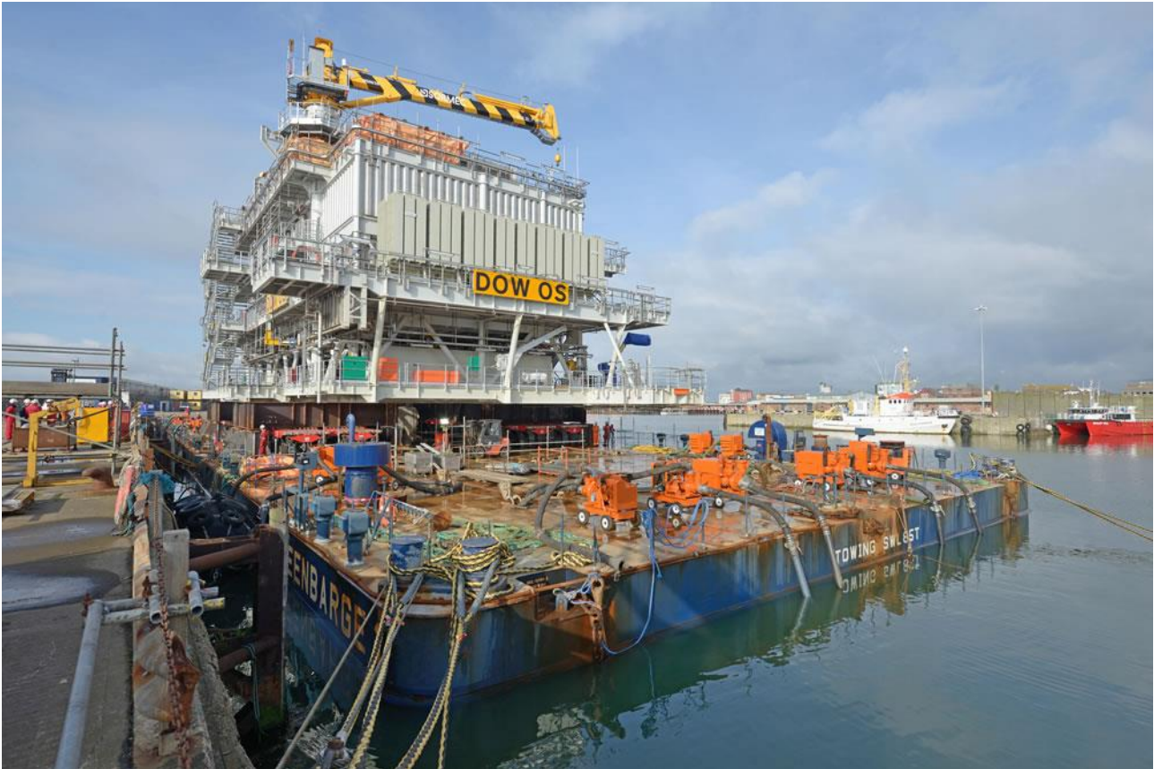
Plate 5-7: Dudgeon OWF OSP being mobilised for installation (Source: Equinor)
