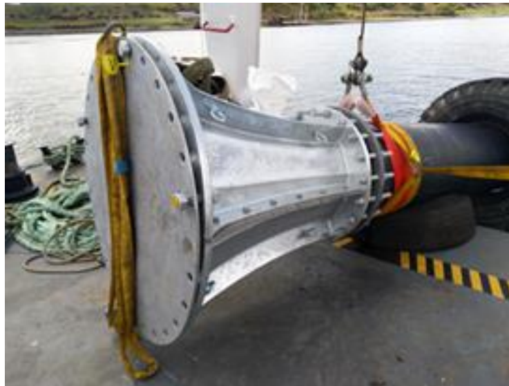
Plate 5-13: Example of bellmouth used to protect the duct ends at the HDD exit point (Source: Equinor)
