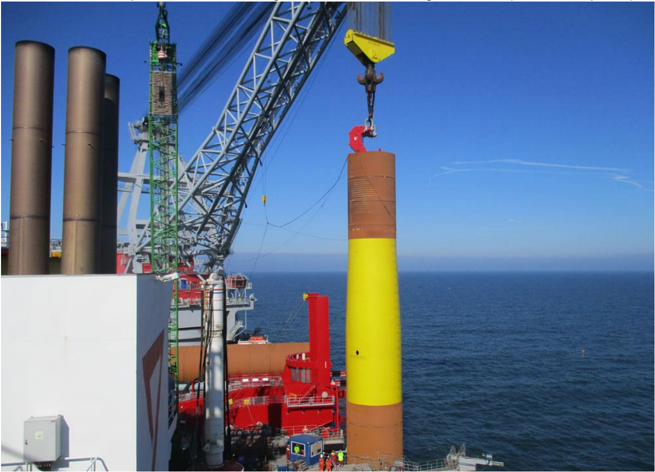
Plate 5-6: Monopile TPs ready for mobilisation to Dudgeon OWF (Source: Equinor)
