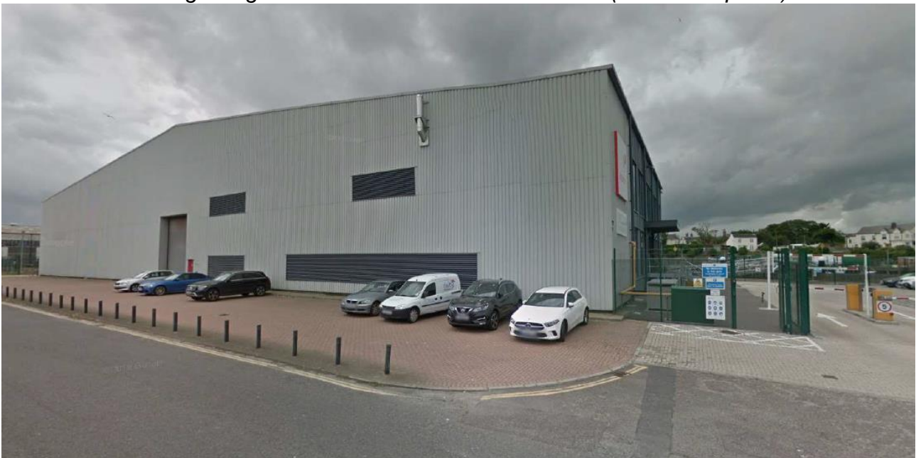
Plate 5-11: Existing Dudgeon O&M base at Great Yarmouth (Source: Equinor)
