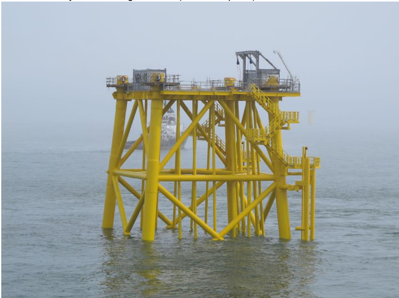
Plate 5-8: OSP jacket at Dudgeon OWF (Source: Equinor)
