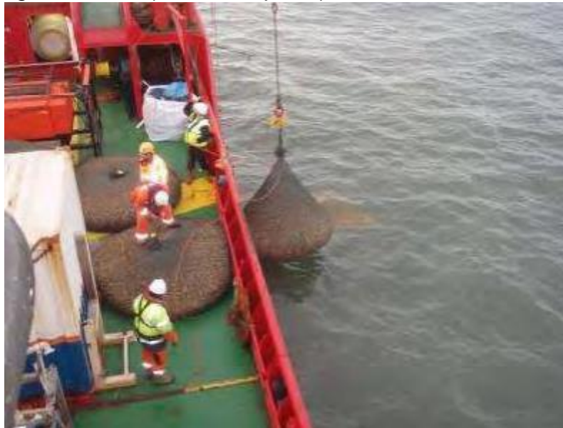
Plate 5-15: Rock bag installation (Source: Equinor)
