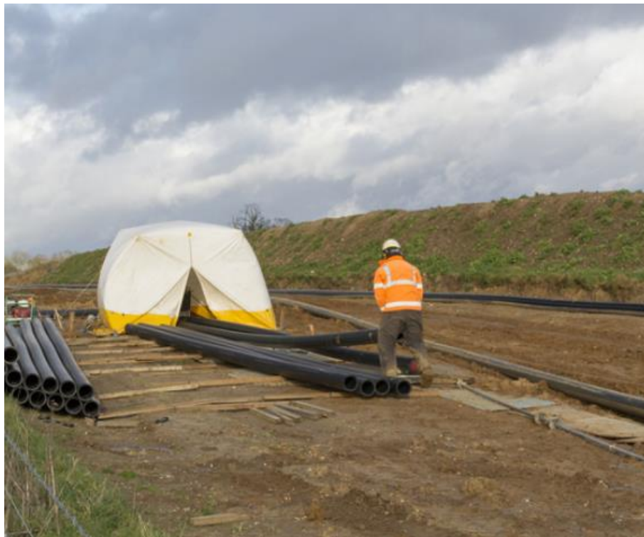
Plate 5-20: Example of hand laying ducts within open trench (Source: Equinor)
