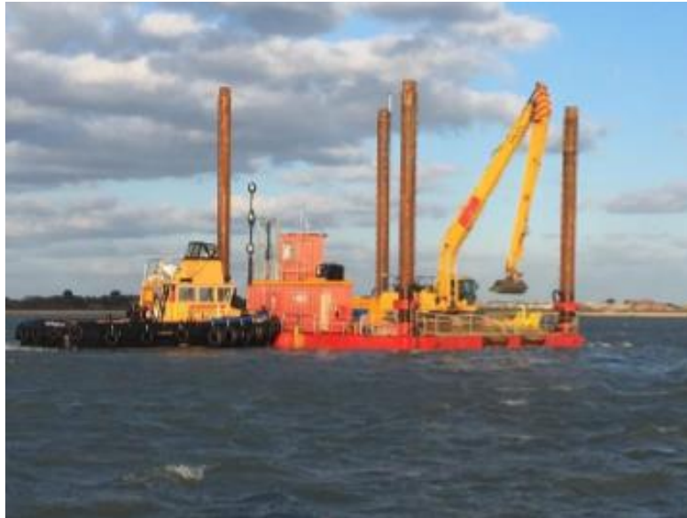
Plate 5-16: Example of a jack-up barge with backhoe excavator (Source: Equinor)
